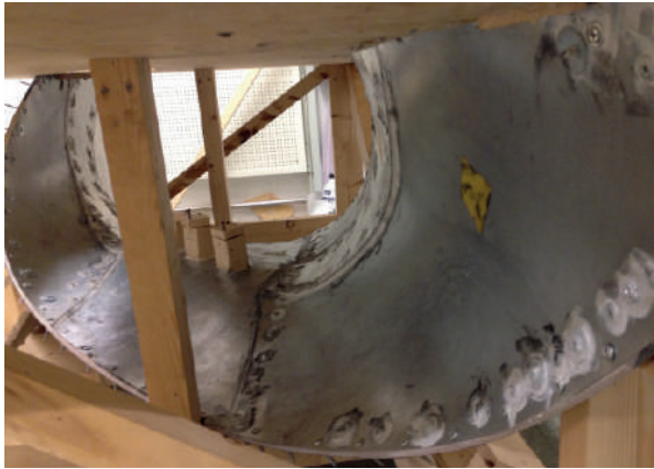
1 Reinforcement and foam border. 2 Inner shell connected with screws, waterproofed. 3 The formwork during casting.
