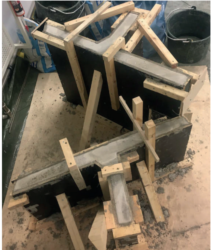
Left side: reinforcement Right side: Formwork after pouring the concrete and adding additional support
