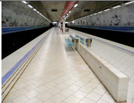
Rissne, well illuminated station, very clean and decorative
