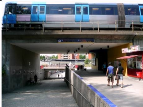
Rågsved, complex structures but with good overview and sight
