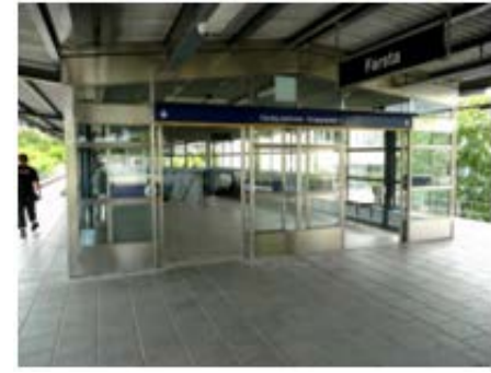
Farsta, glassed transition area; good sight from and to platform
